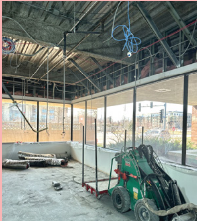
Waiting Room in Progress
