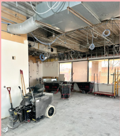
Waiting Room in Progress
