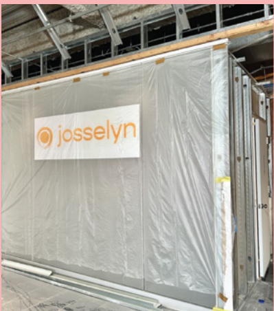
Reception Desk Area in Progress
